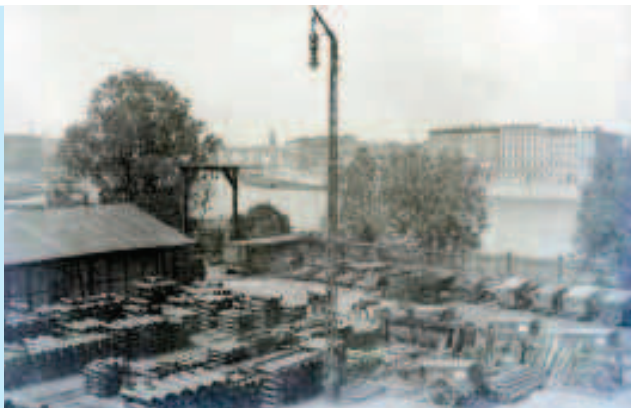
[71] Wrocław. Magazyn rur (arch. MPWiK Wrocław)
